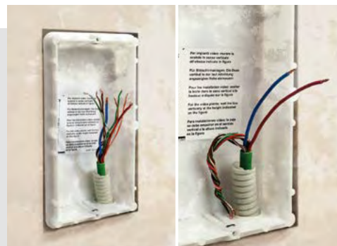
Remove the old entrance panel being replaced.
