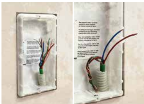
Remove the old entrance panel.
