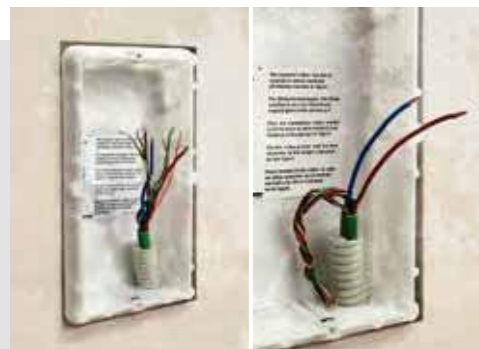
Remove the old entrance panel being replaced.
